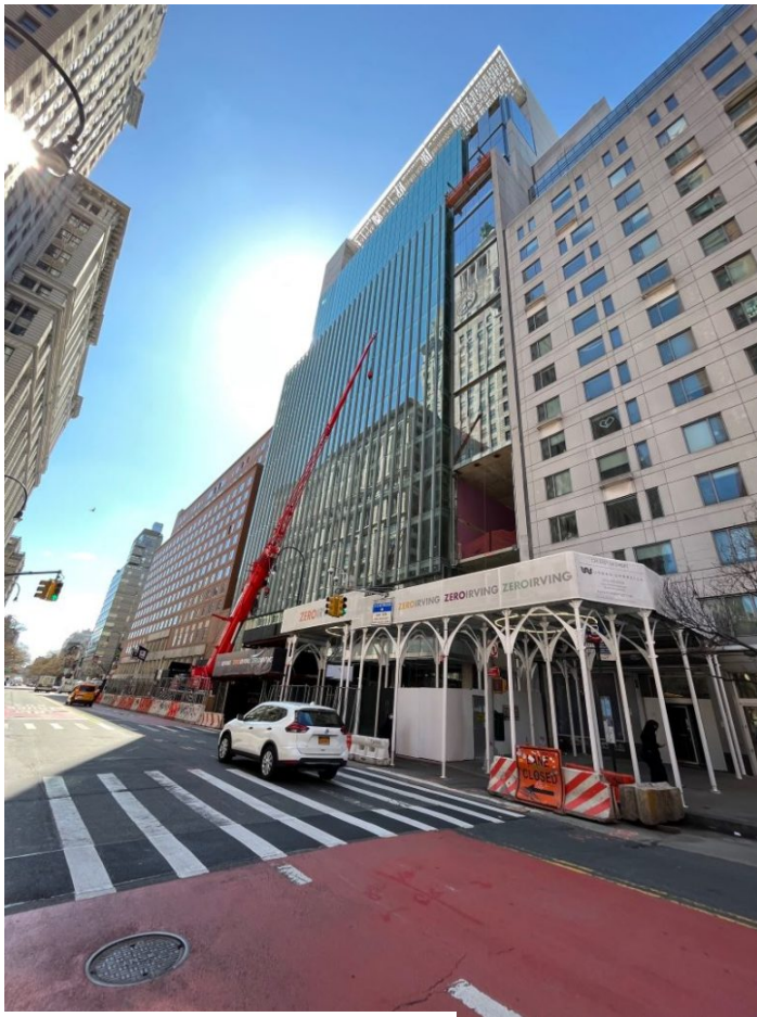
View of construction at Zero Irving
