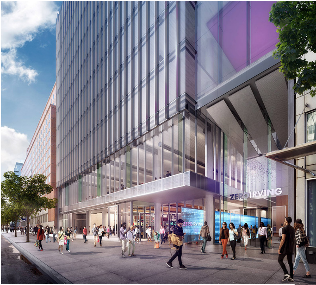
Entry at Zero Irving Roof Terrace at Zero Irving (Courtesy of Davis Brody Bond)
