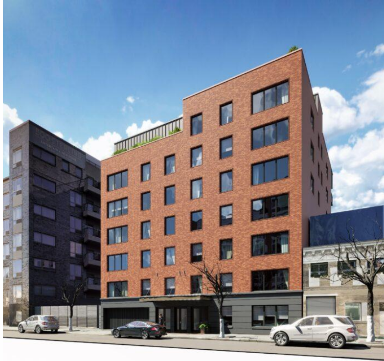
488 Sterling Place is a luxury eco-friendly development three blocks from Prospect Park / ©Travis Mark
