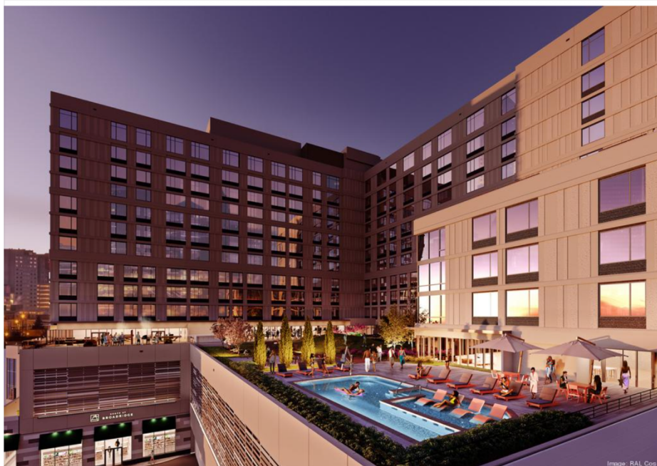
An expansive outdoor amenity area on the fourth floor.
