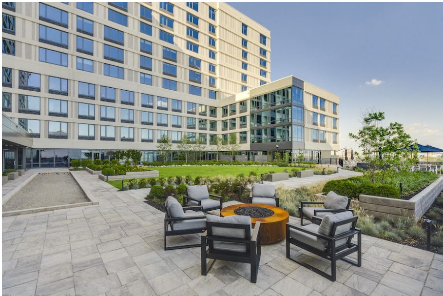
The 476-unit Broadridge, which welcomed its first tenants this fall, is the largest one-building rental apartment community in the city. | Photo courtesy RAL Properties
