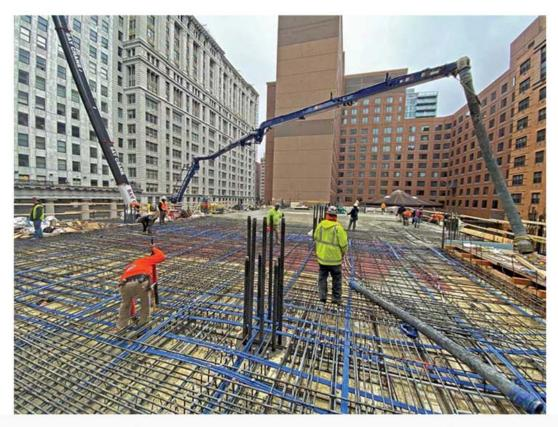
Workers place concrete for the third floor of Zero Irving, a 21-story posttension concrete structure that will house tech companies. PHOTO BY RAL COS.
